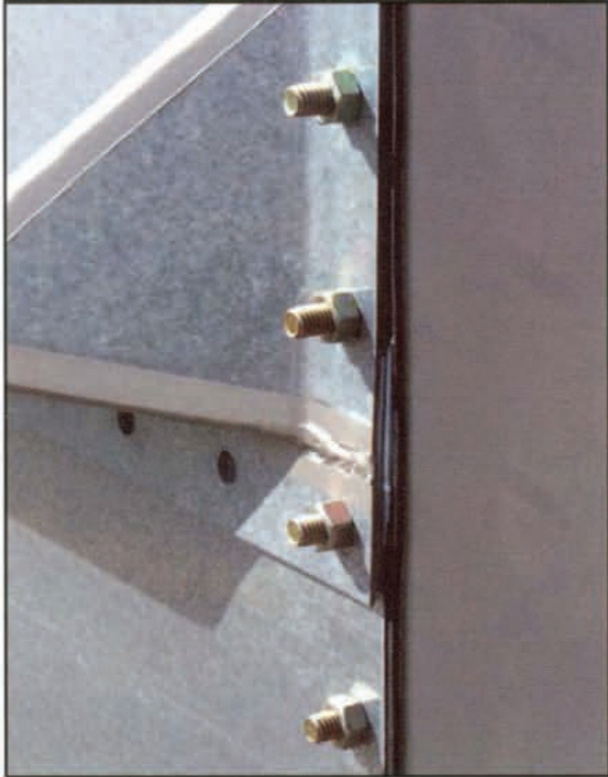
CONNECTION WITH CAULKING
