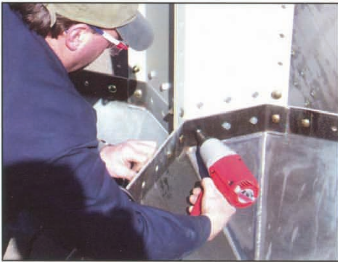
Tightening of the three self-tapping bolts into the hopper starter strip.
