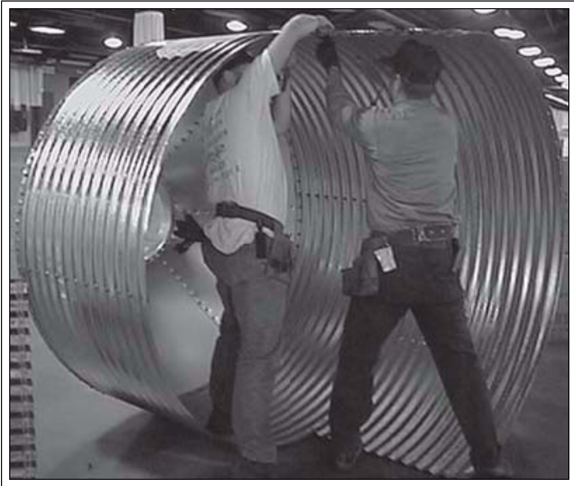
Figure 6F Sidewall Assembly
