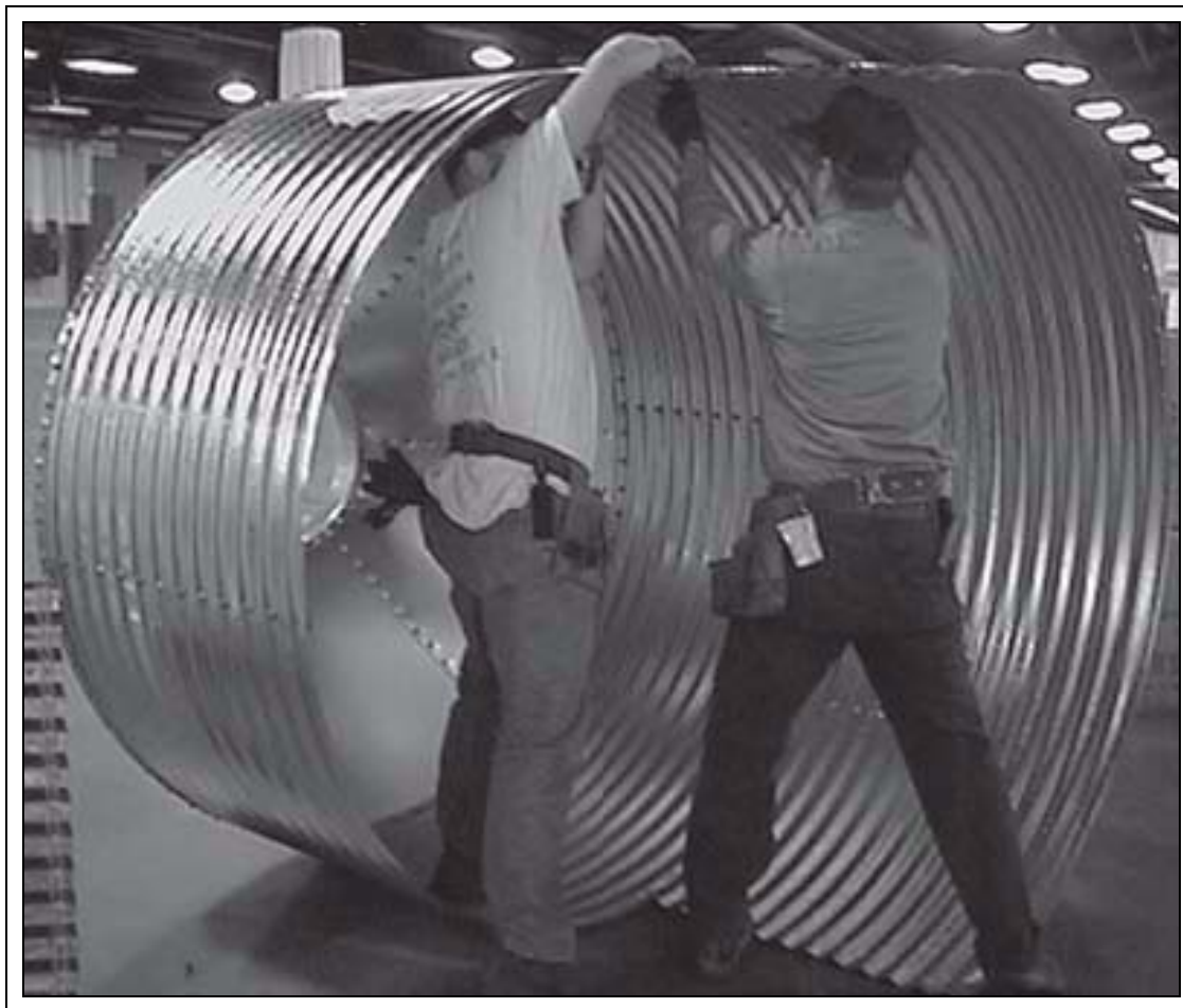
Figure 6F Sidewall Assembly
