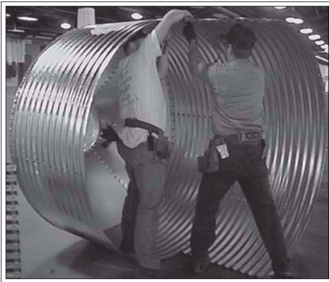
Figure 6F Sidewall Assembly
