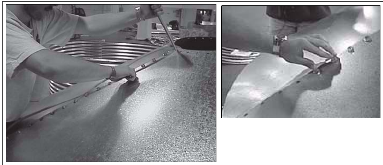
Figure 7B Lining Up Holes and Placing Bolts
