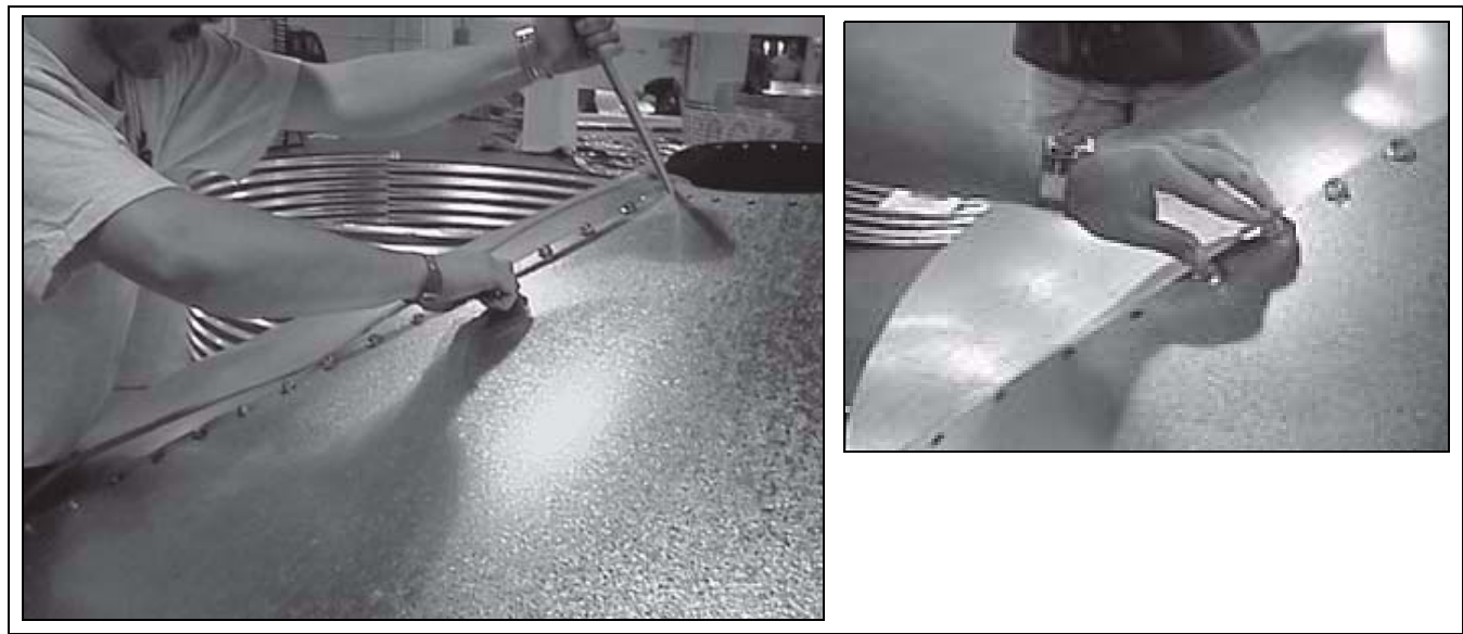
Figure 7B Lining Up Holes and Placing Bolts
