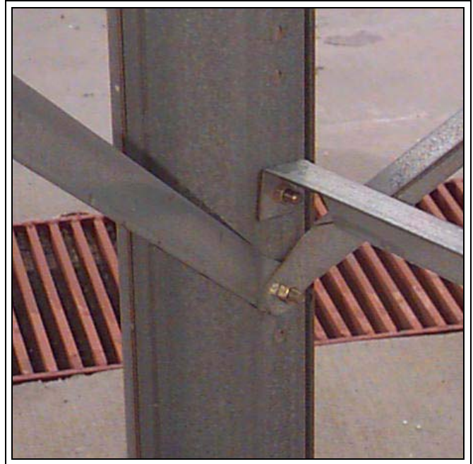
Figure 12H Brace to Leg Connection
