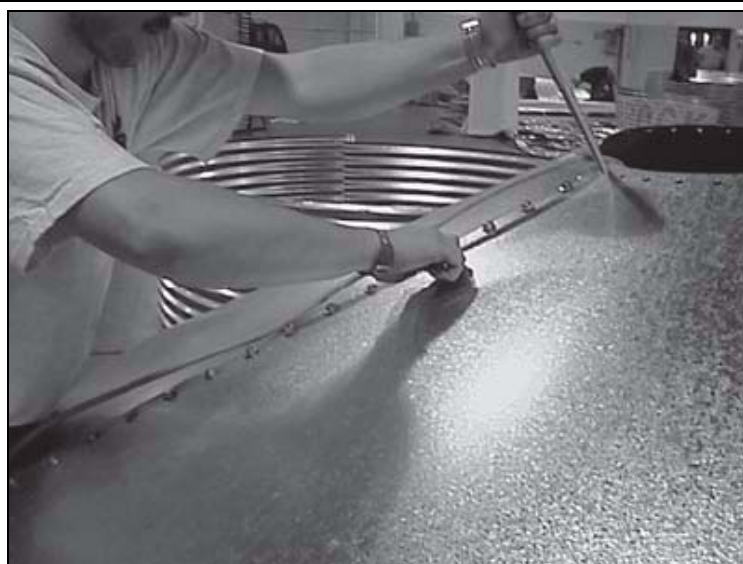
Figure 7B Lining Up Holes and Placing Bolts
