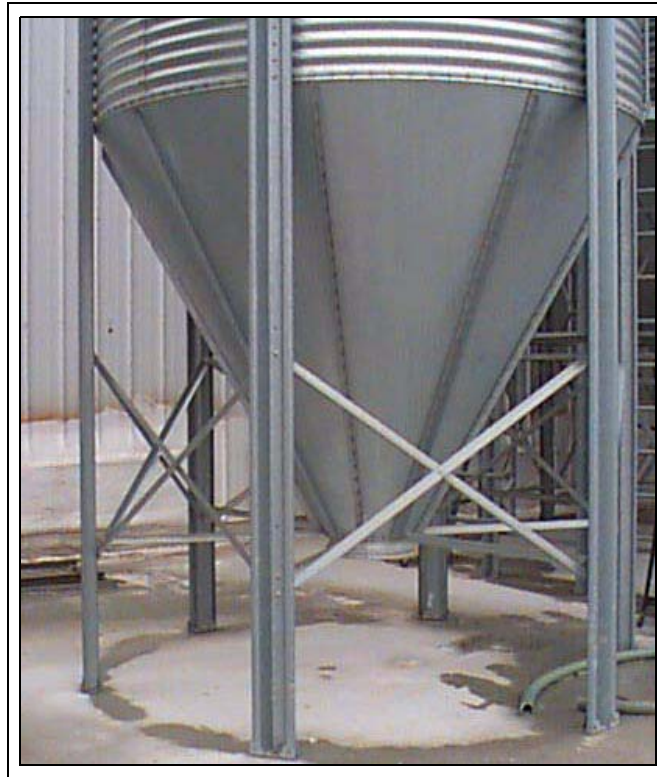
Figure 12F 1 Set of Cross Tie Braces
