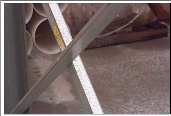
Figure 12G Cross Tie to Cross Tie Connection
