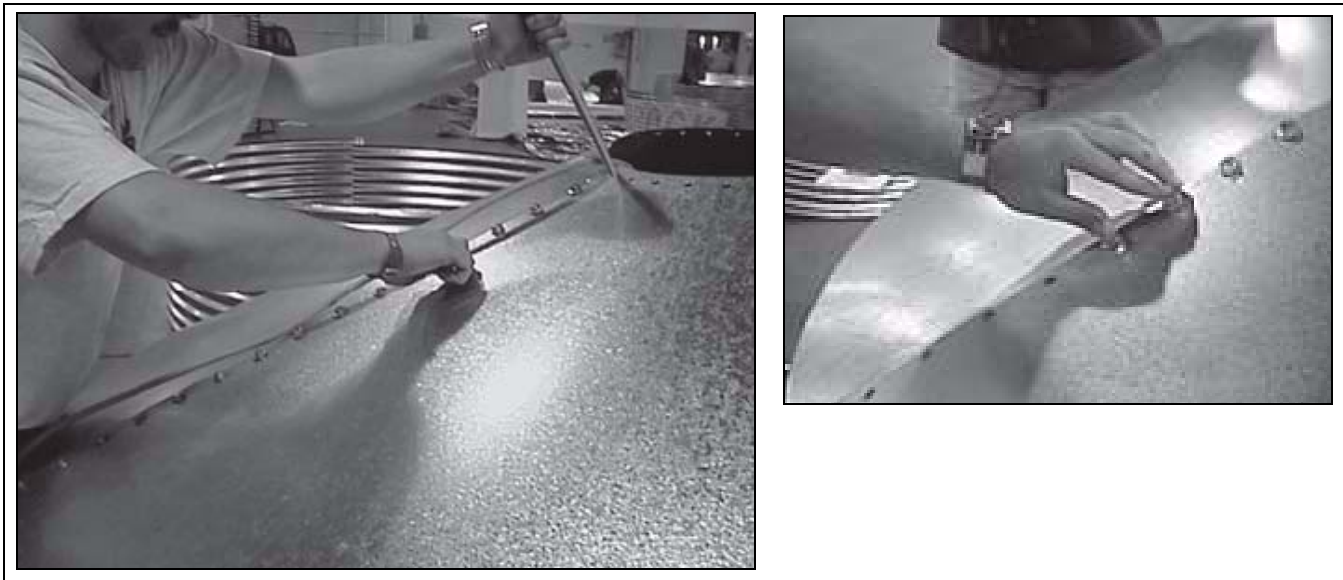
Figure 7B Lining Up Holes and Placing Bolts
