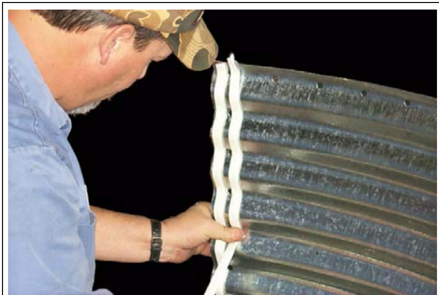
Caulking is applied to all BFT parts before assembly.
