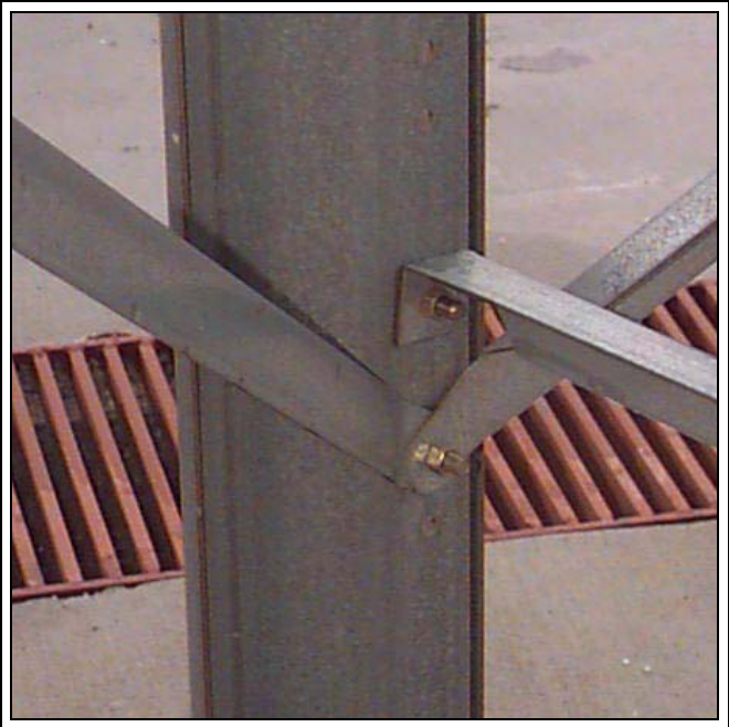
Figure 13H Brace to Leg Connection
