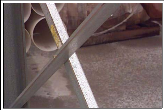
Figure 13G Cross Tie to Cross Tie Connection
