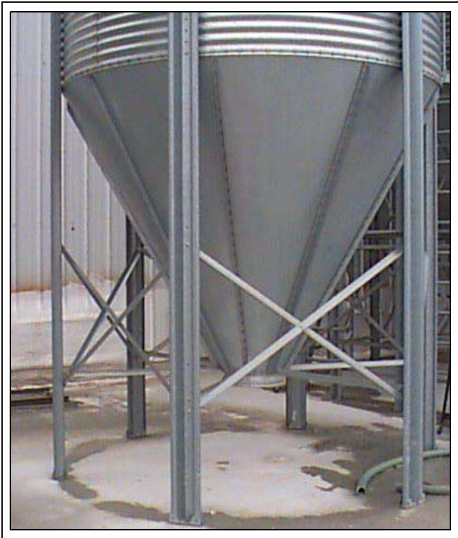
Figure 13F 1 Set of Cross Tie Braces
