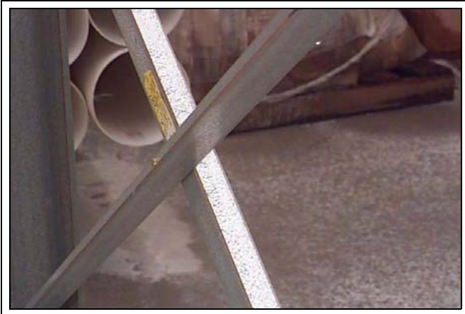
Figure 13G Cross Tie to Cross Tie Connection
