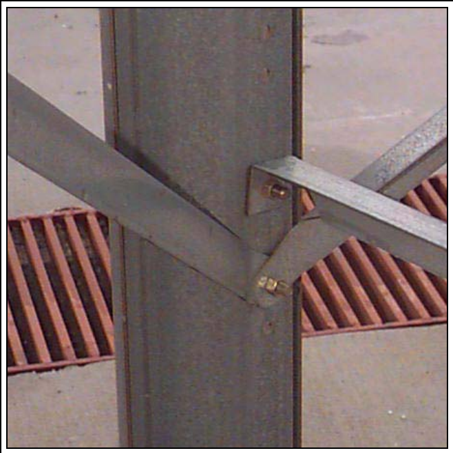
Figure 13H Brace to Leg Connection
