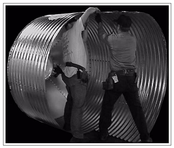
Figure 6F Sidewall Assembly
