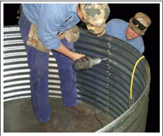
First ring assembly. Tighten bolts from the nut side only.
