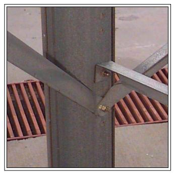
Figure 13H Brace to Leg Connection
