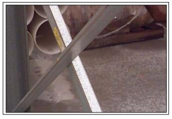
Figure 13G Cross Tie to Cross Tie Connection
