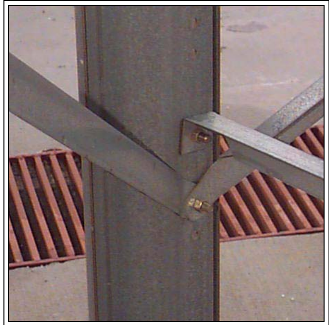
Figure 12H Brace to Leg Connection
