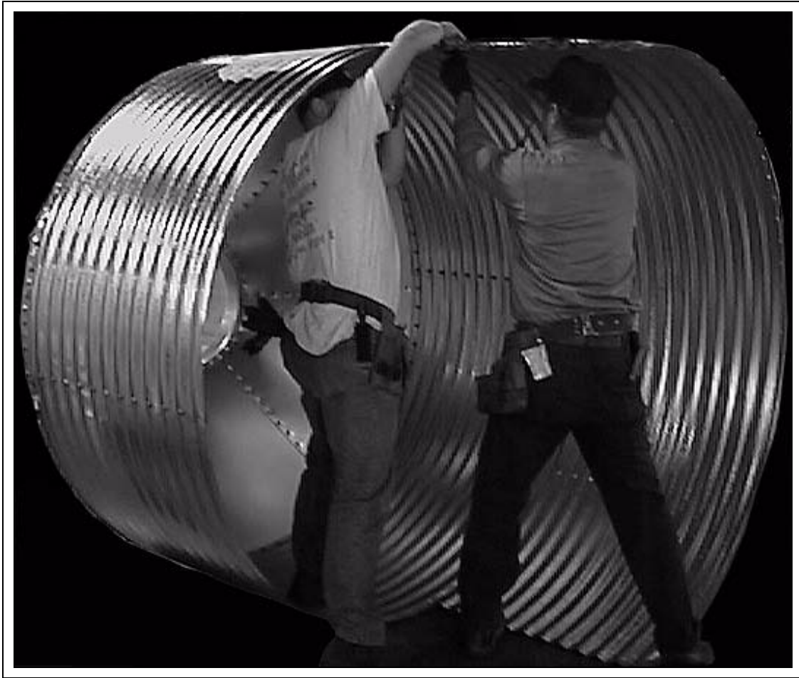
Figure 6F Sidewall Assembly
