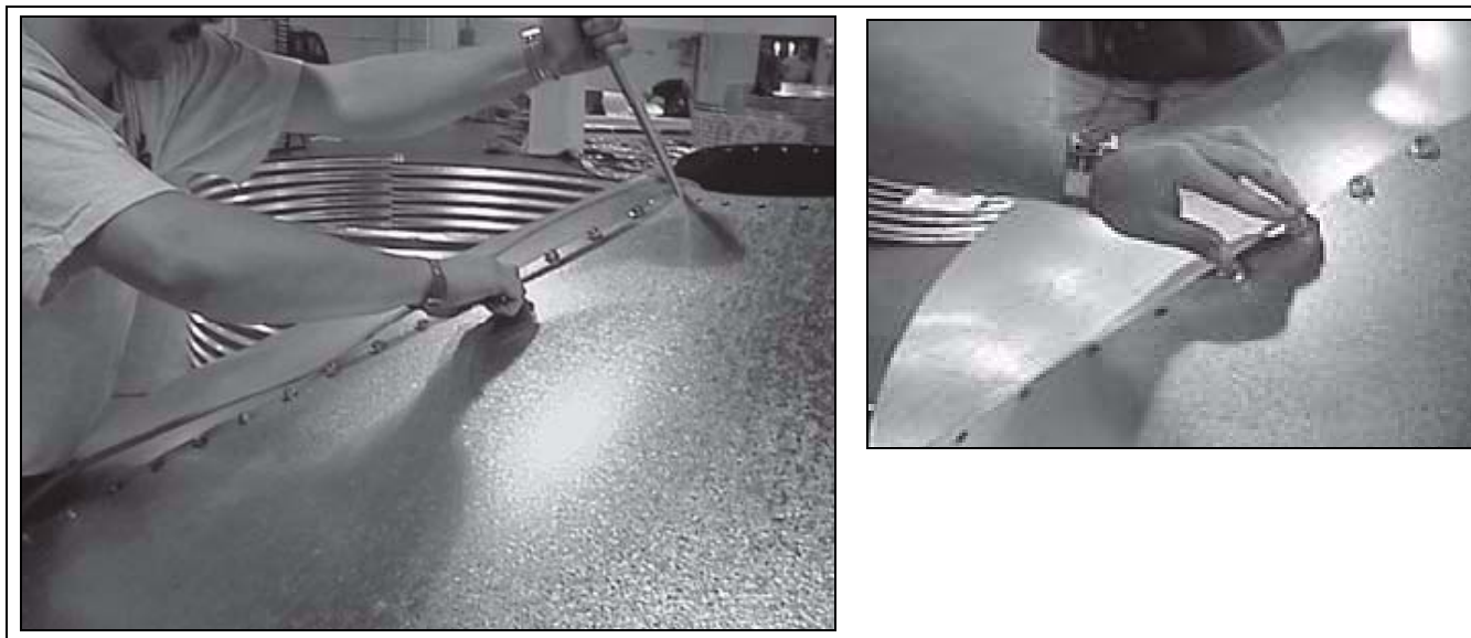
Figure 7B Lining Up Holes and Placing Bolts
