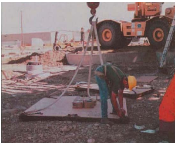
Installing erection platforms (supplied by contractor)
