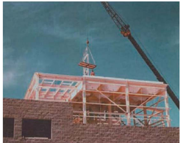
Installing erection platforms (supplied by contractor)
