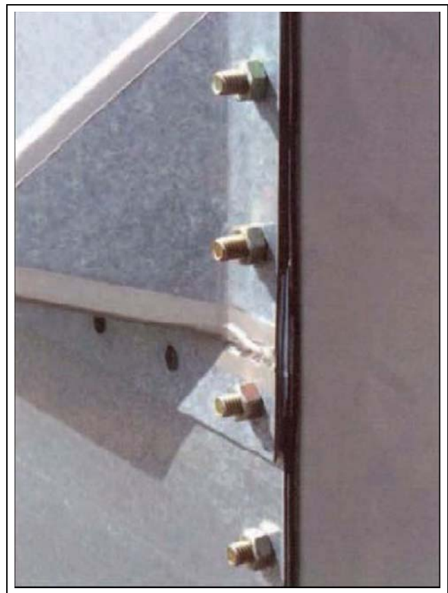
Figure 2AB Connection with Caulking
