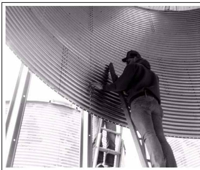
Figure 9H Installing legs to bin with bolt heads on the inside of bin and nuts on the outside.
