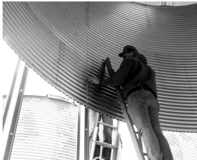
Figure 2: Installing legs to bin with bolt heads on the inside of bin and nuts on the outside.
