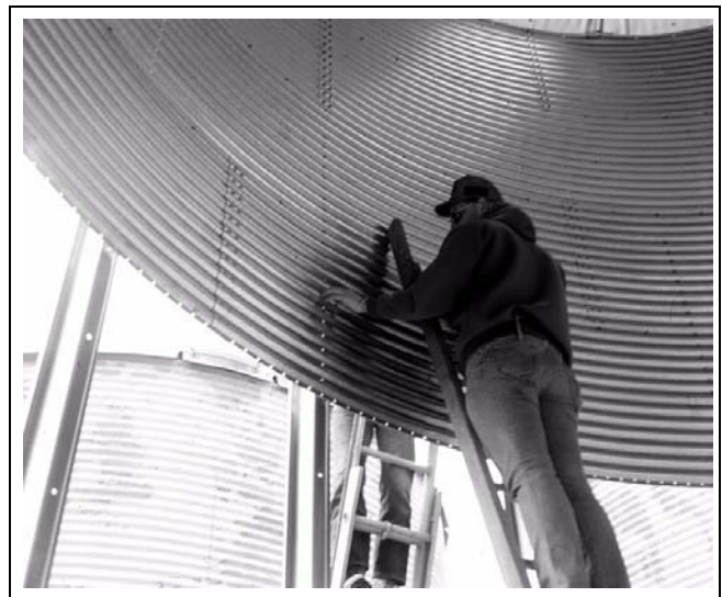
Figure 9H Installing legs to bin with bolt heads on the inside of bin and nuts on the outside.
