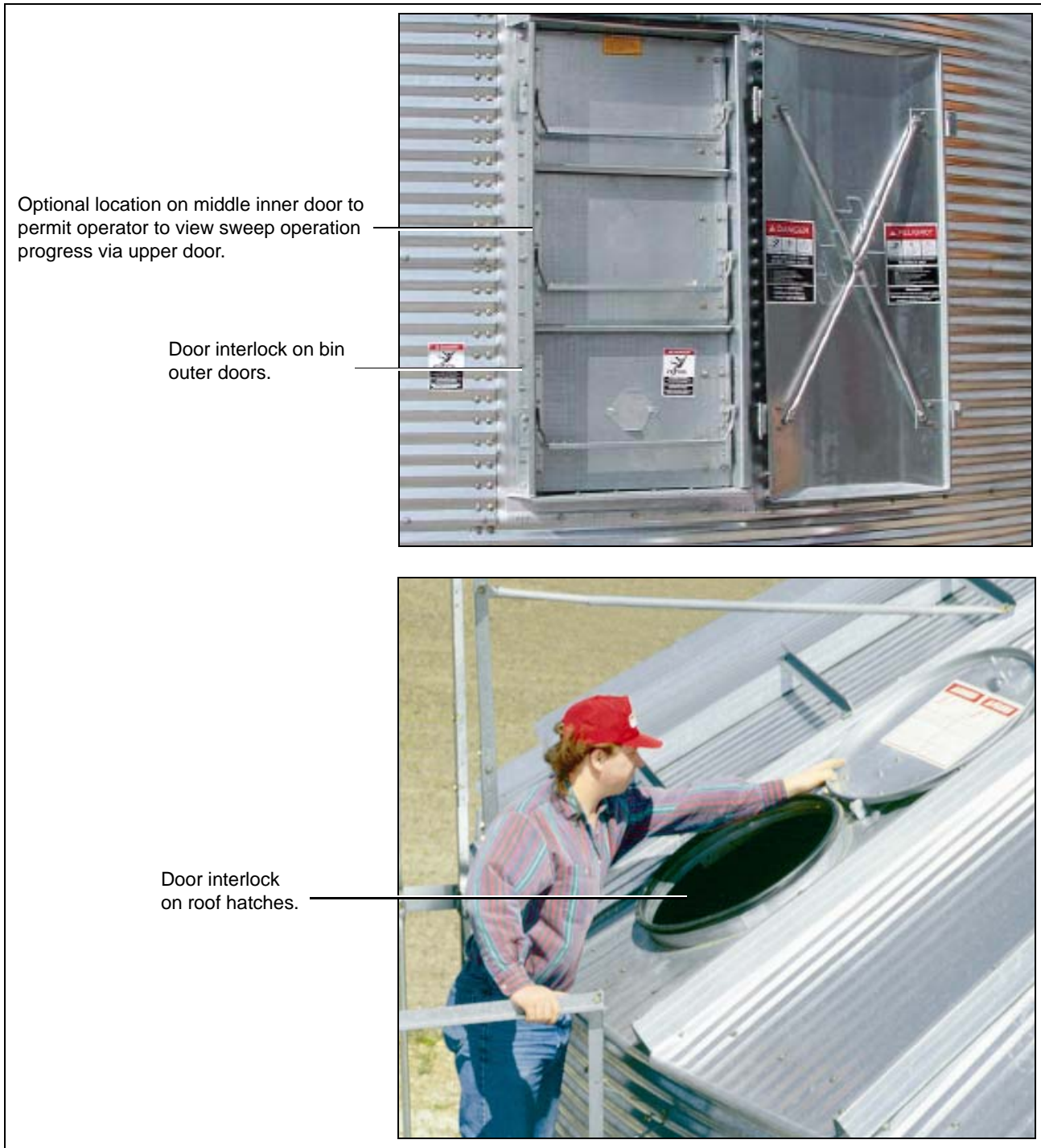
Figure 5A Door Interlock Switch Locations
