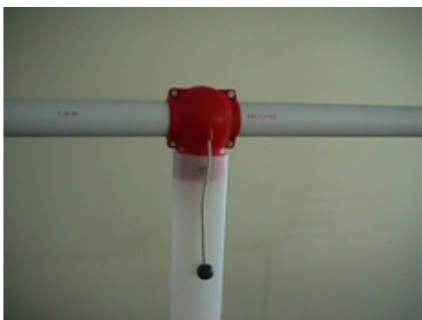
Figure 14: Drop Kit installation w/ Drop Tube
