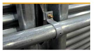
Wind ring and bracket design reduces bolt holes in stiffeners, resulting in increased load capacity.
